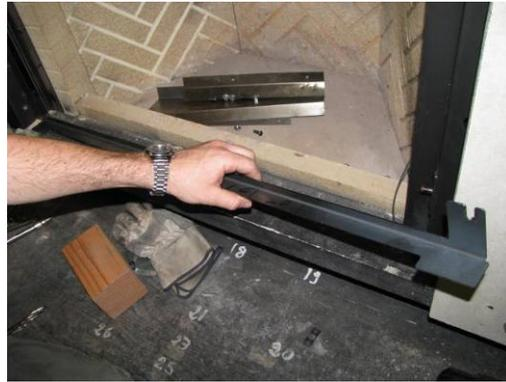
**You can stop here if you only want to change the stainless steel gasket at the bottom of the guillotine frame.**
