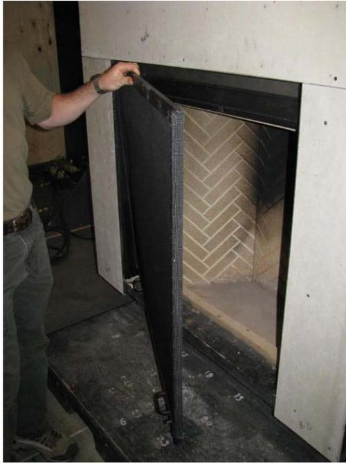
**You can stop here if you only want to change the gasket on the firescreen to ease its sliding up and down.**
